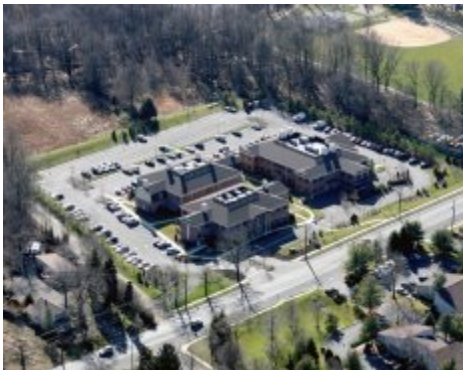
Warren Office Center, Warren, NJ
